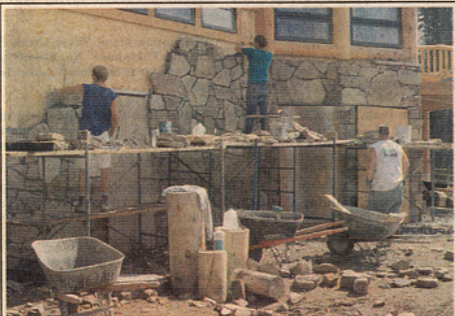
STONEMAN — Rick Demarest, pictured above right on the scaffolding, and his crew work on the exterior of the Patch home, which overall will probably consist of more than 40 tons of rock and stone.
